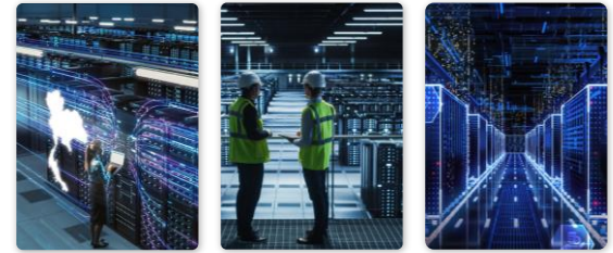
Data Service Installation Data Center
